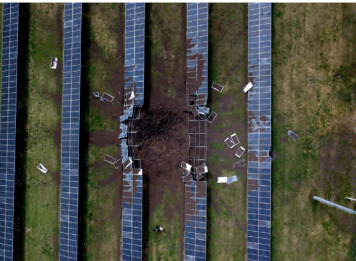
Russian attacks damaged a number of solar power panels at a station in Merefa, on the outskirts of Kharkiv, in May 2022.
