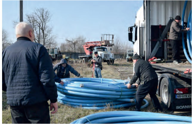
Teltow has mobilized relief worth hundreds of thousands of euros, via funding projects and private donors, to assist the reconstruction.
